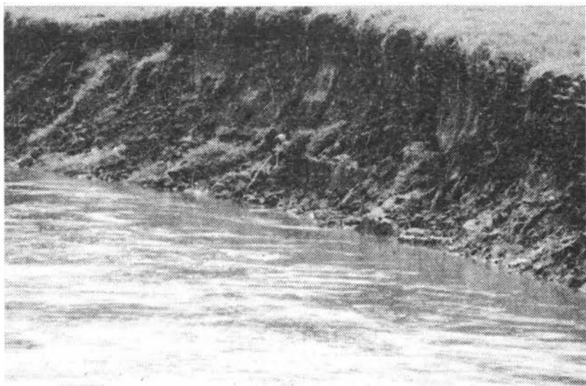
Figure 5 Severe riverbank erosion along meander bend C' caused by the extreme discharge during tropical cyclone Gavin in March 1997. For scale, note the woman fishing in the centre of the photograph.
